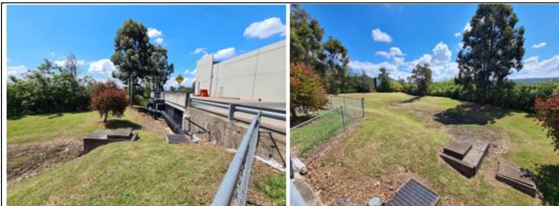
Detention basin and vegetation on site
