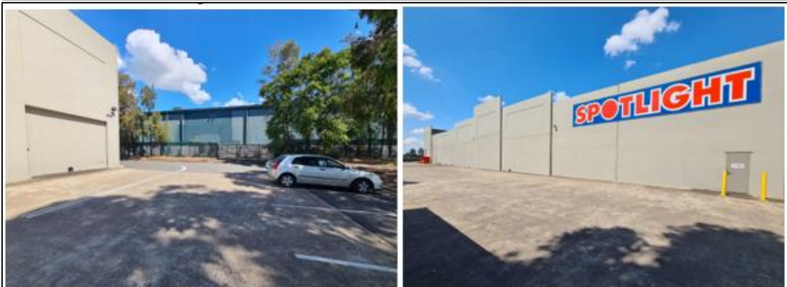
Existing hardstand - Proposed extension area
